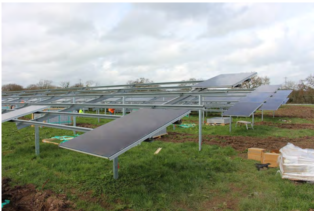
Plate 10: Mounting of PV modules
