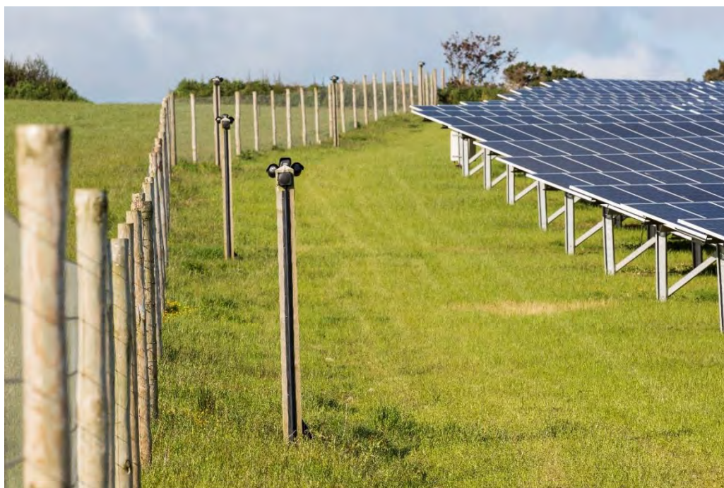
Plate 4: Example of security fencing and monitoring cameras
