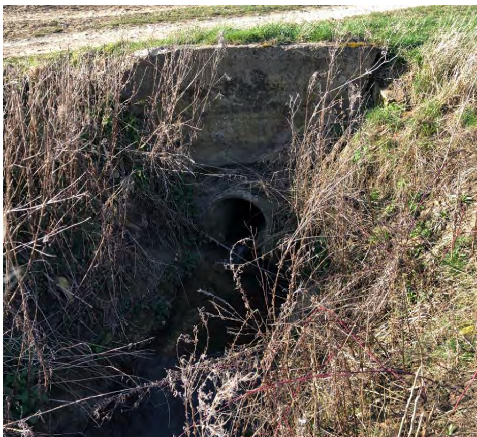
Plate 12.2: Watercourse Crossings within the Site (Land Drain at E 505939, N 312244)
