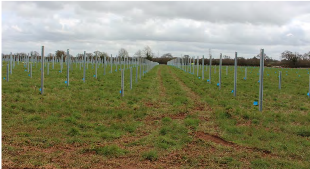
Plate 9b: Installation of PV module mounting structures (2 of 4)
