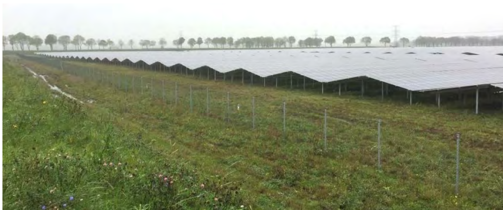
Plate 1 - Example of East West Configuration
