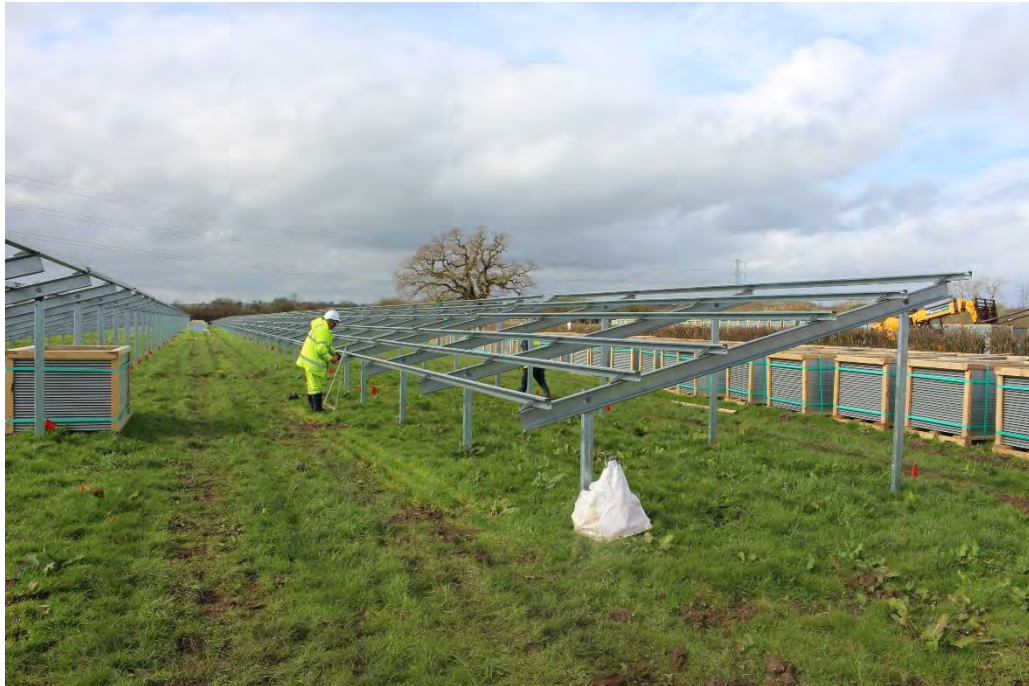
Plate 9d: Installation of PV module mounting structures (4 of 4)
