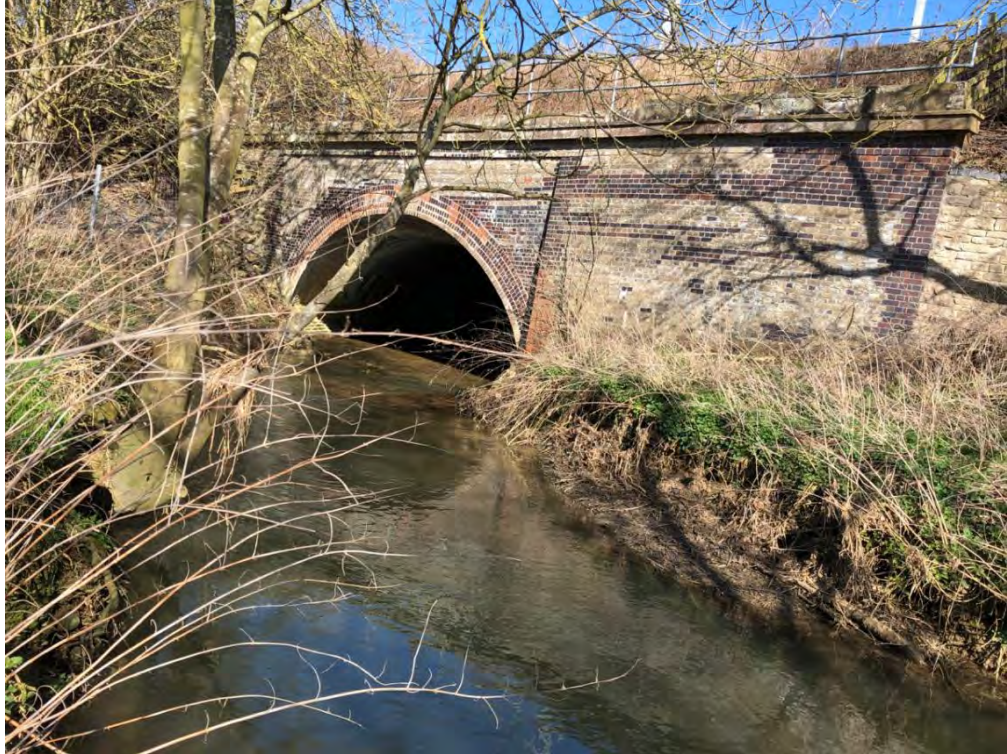
Plate 12.1: Watercourse Crossings within the Site (West Glen River at E 504909, N 312076)
