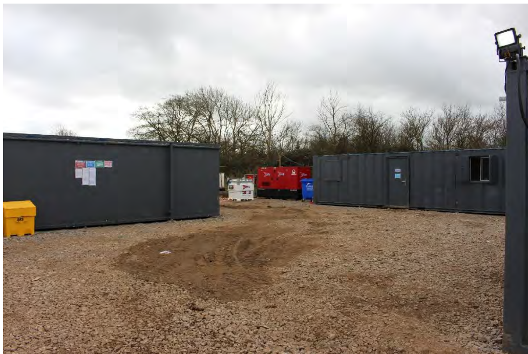
Plate 7: Establishment of the temporary construction compound(s)
