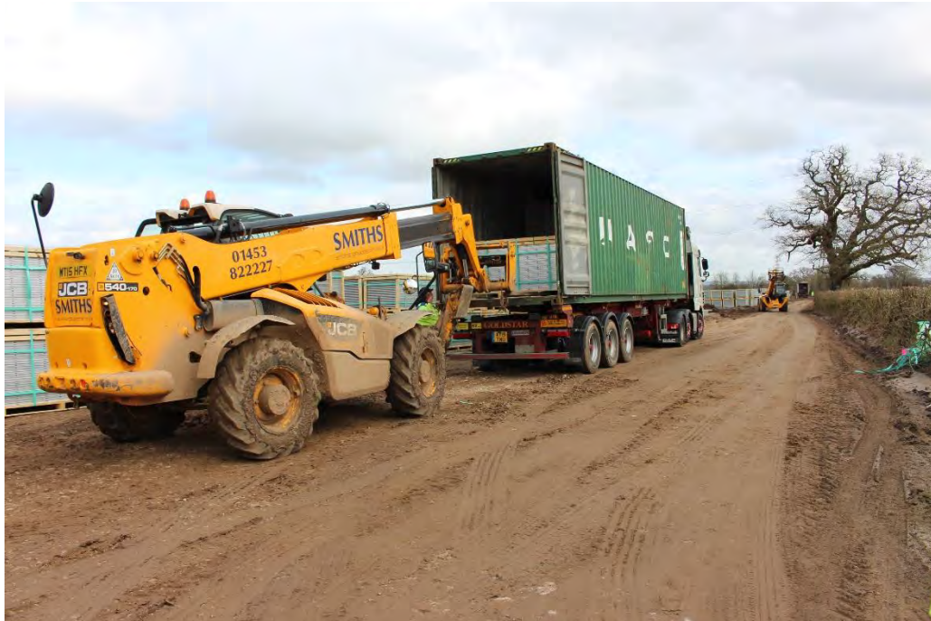
Plate 5: Delivery of construction materials, plant and equipment to Site
