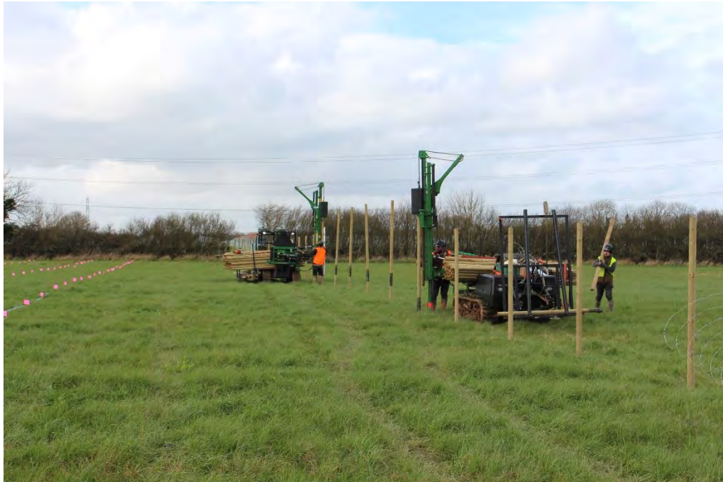
Plate 6: Establishment of Site fencing
