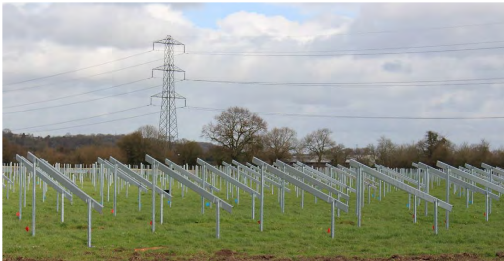
Plate 9c: Installation of PV module mounting structures (3 of 4)
