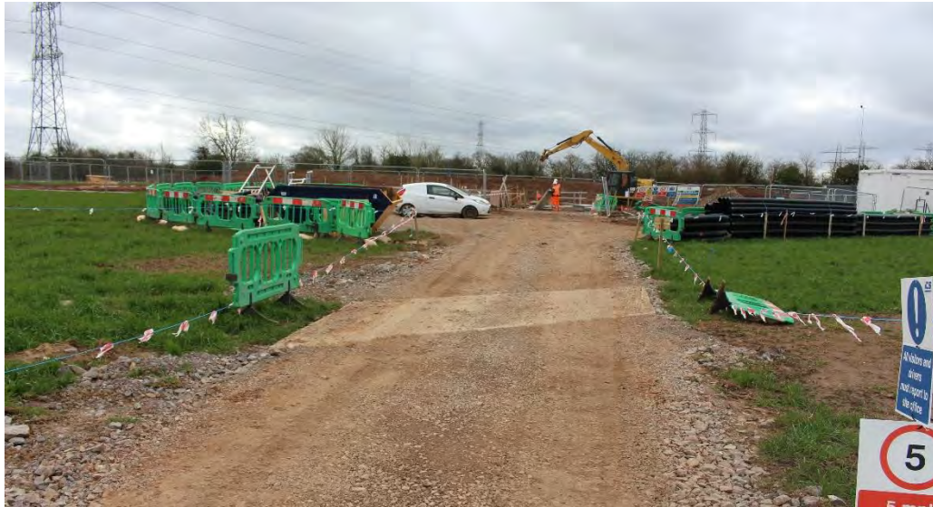
Plate 8: Establishment of internal access tracks and crossing of underground utilities
