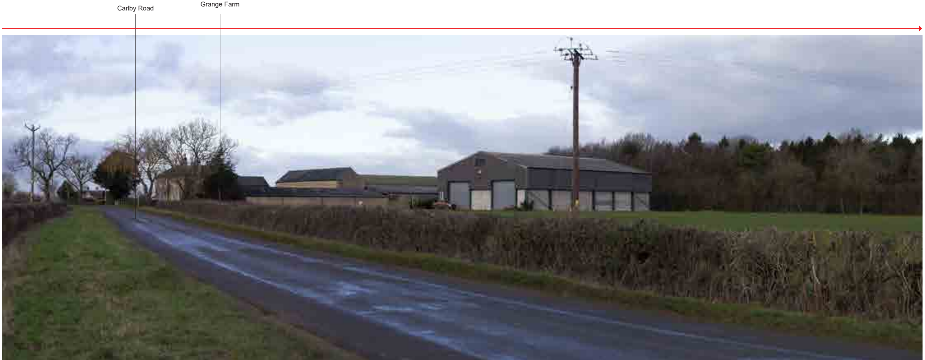
Representative Viewpoint 5 (Right) - Carlby Road, East of Braceborough Grange
