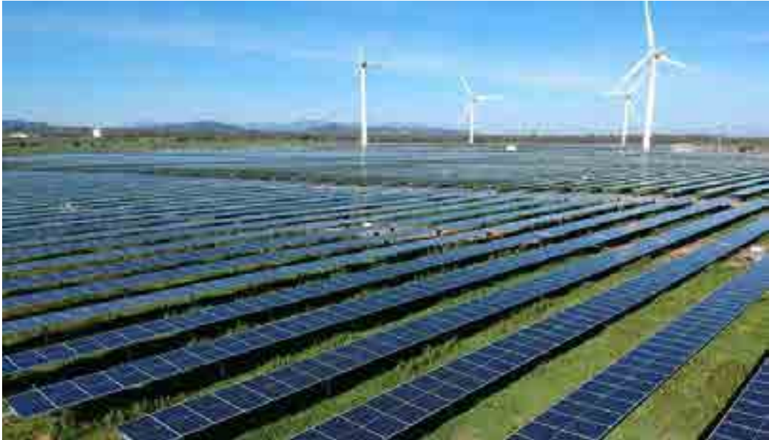
Plate 2: Single Axis Tracker Arrays
