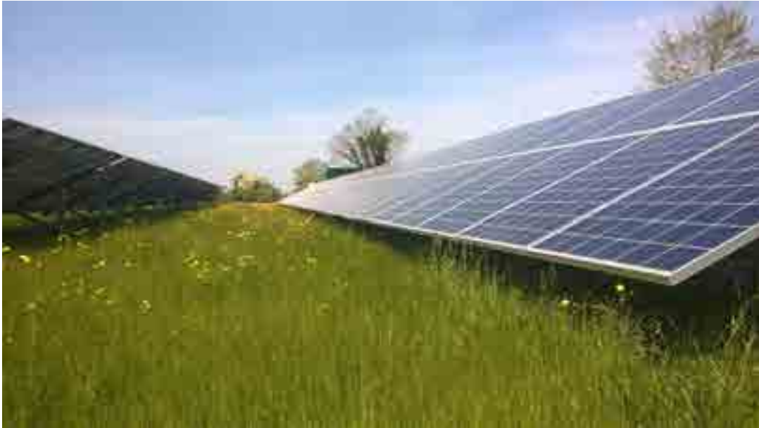
Plate 1: Fixed South Facing Arrays
